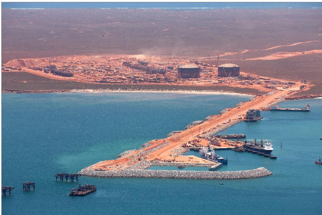
An aerial view of the foundation structures for the LNG jetty and the materials offloading facility on Barrow Island looking back towards the plant site.
